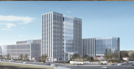
Beijing Headquarter (under construction)
